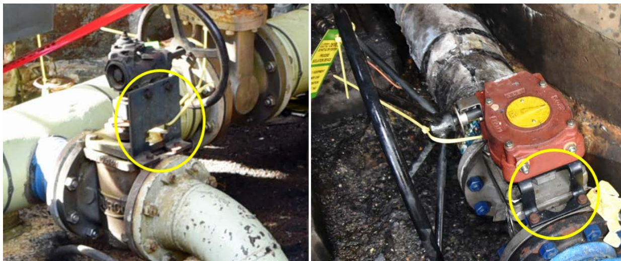
Figure 8. Two of several designs of gearbox support brackets (yellow circles) used at the Baton Rouge refinery. These specific brackets attach to the valve body flange – they are not among the approximately three percent of valves in the alkylation unit that attach the gearbox support bracket using the same four vertical bolts that secure the pressure-retaining top-cap.
